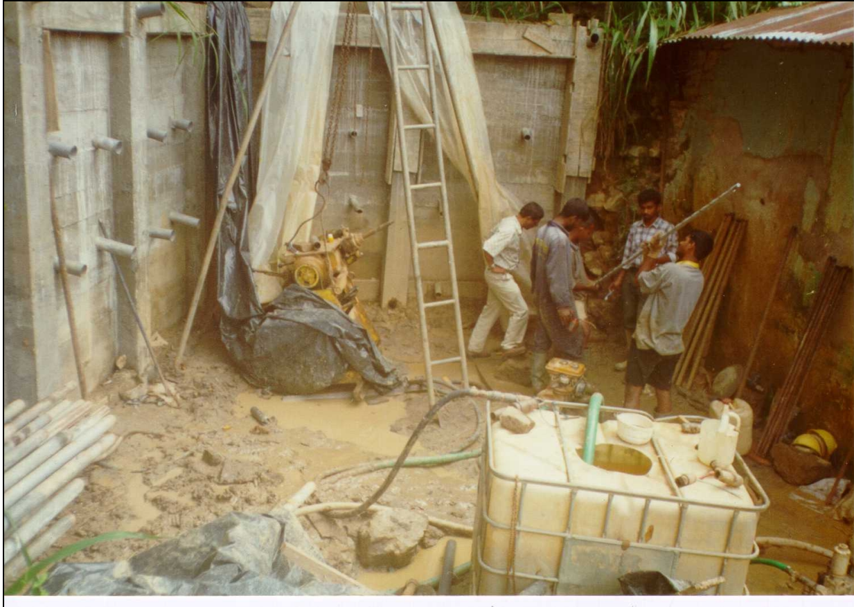
Fig. 2. Photograph showing soil nailing through a simple retaining structure. The structure supports the earth slip over peaty clay soil to the right of the photo. Weep holes drains excess water in the disturbed soil mass
