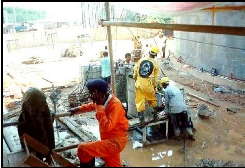
Fig. 4. Grouting operation under petroleum storage tanks in the marshy lands at Orugodawatta, Colombo.
